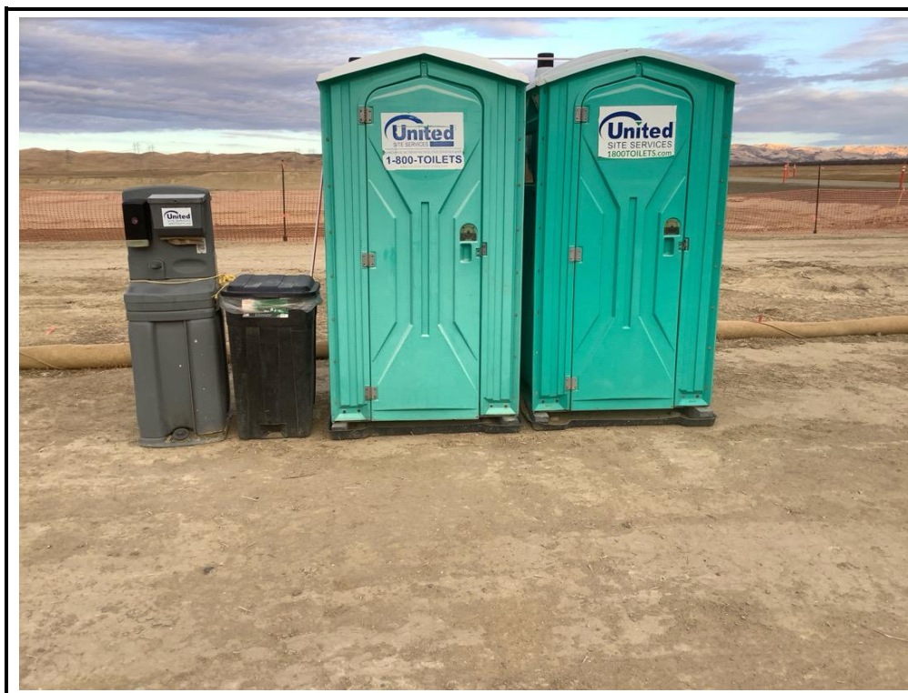
Photograph 6: Bathrooms and wash station secured with secondary containment on 5/4/2026.
