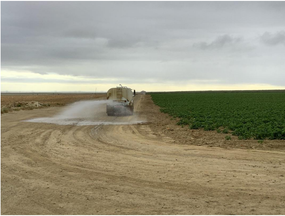
Photograph 1: A water truck spraying water along the access road on 4/2/2026.
