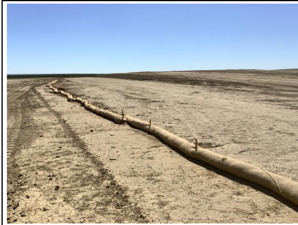
Photograph 3: BMPs in working order on 4/14/2026.
