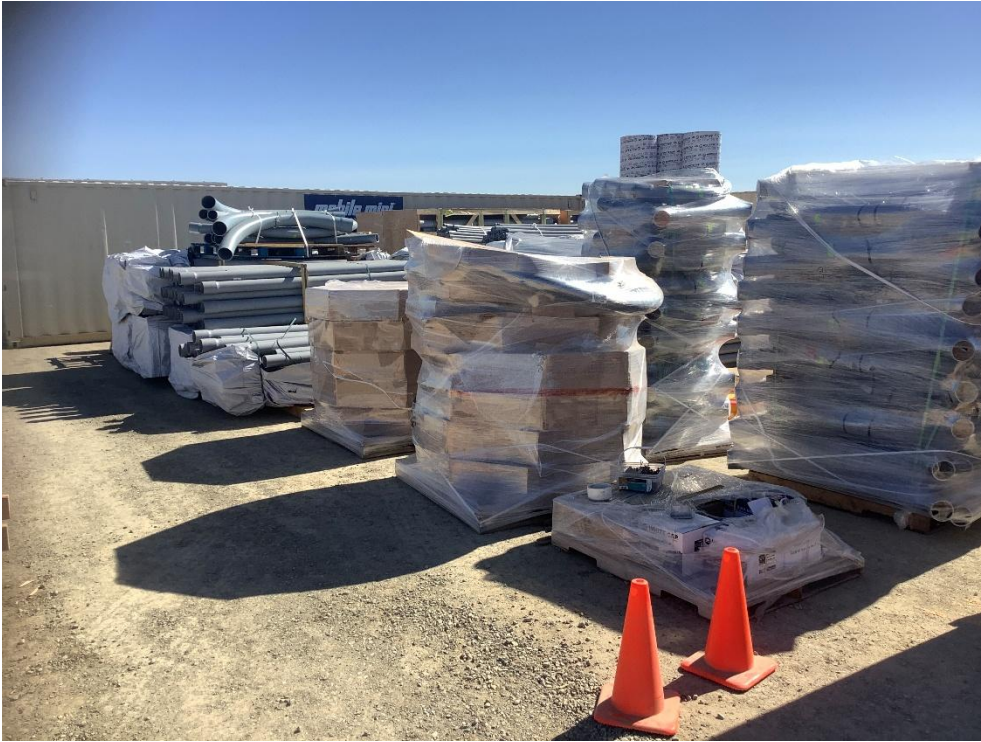
Photograph 11: Materials staged on site on 6/19/2026.
