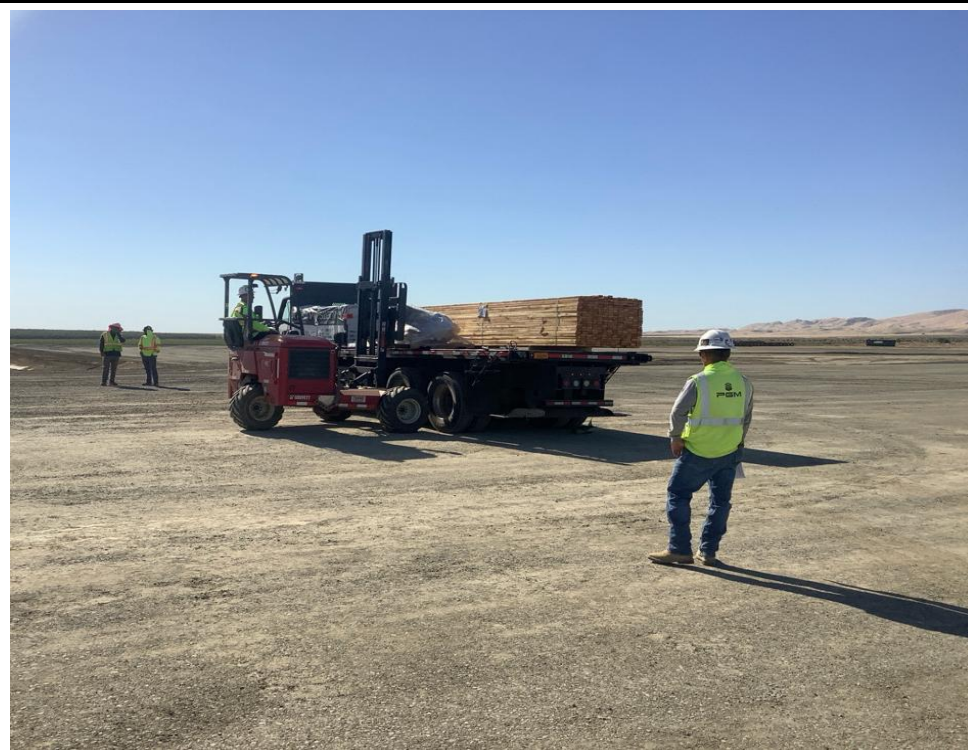
Photograph 10: Crews unloaded and staged materials on site on 6/15/2026.
